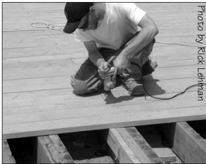
Construction of Long Branch, NJ's recycled plastic lumber boardwalk.
