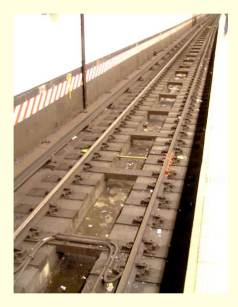
The newer subway track ties installed by MTA/NYC Transit are also ekki.
